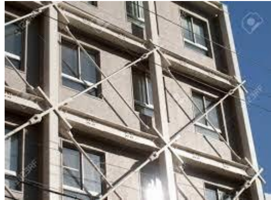
Fig 14.2 seismic retrofitting
